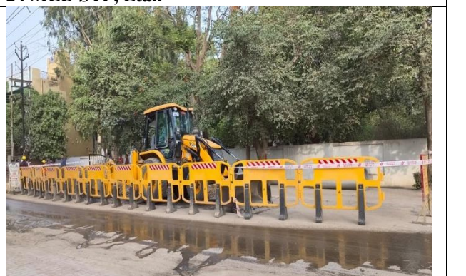
Sewer Laying, Mirzapur
