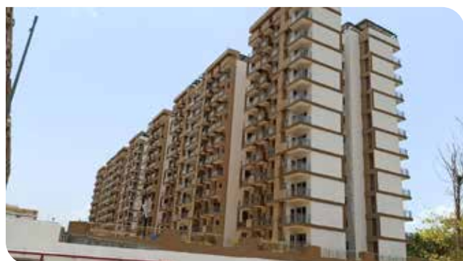
CPWD RBI Building Work, Mumbai
