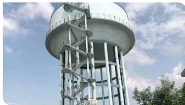
80 MLD Water Treatment Plant, Unnao
