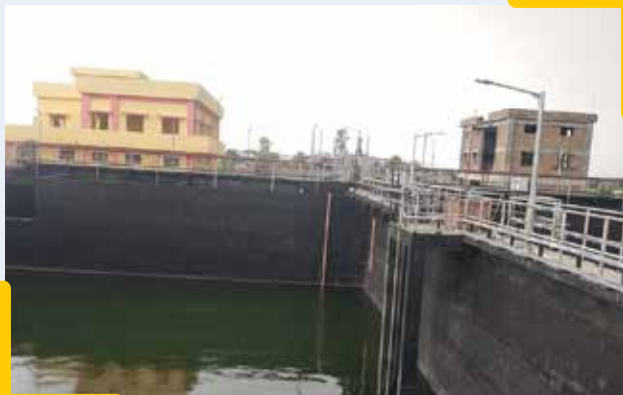
Hanumangarh Sewerage Work (Rajasthan)
