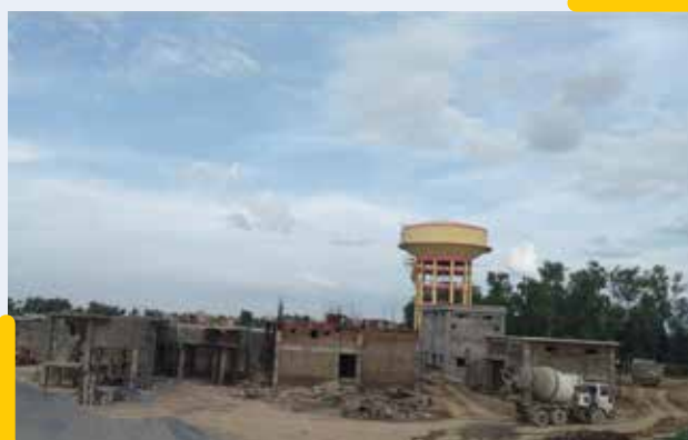
Hanumangarh Sewerage Work (Rajasthan)
