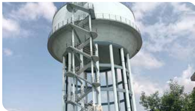
80 MLD Water Treatment Plant, Unnao
