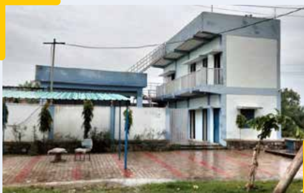
Sewerage Network, Raipur (Dehradun)
