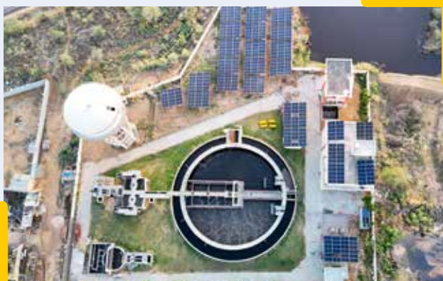
4.5 MLD STP, Sikar (Rajasthan)
