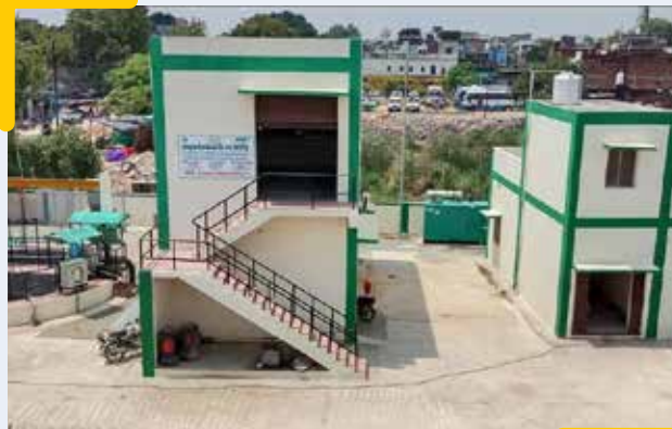
Mirzapur Pumping Station
