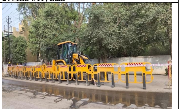
Sewer Laying, Mirzapur
